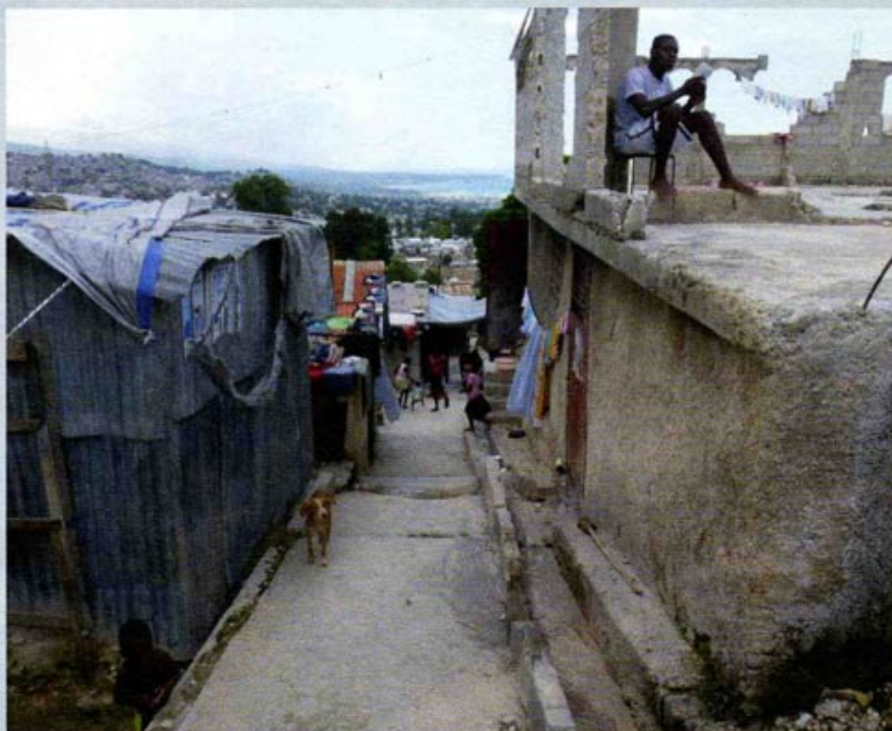
View of the district of Baillergeau, Haiti.
