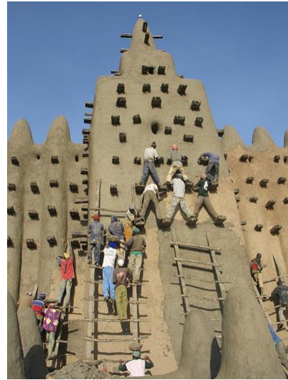
Replastering of the Great Mosque of Djenné, Mali, during the 10th International Conference on the Study and Conservation of Earthen Architectural Heritage, 2008
